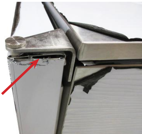
Minor door damage close-up
