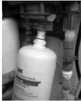
Remove red sanitary cap from RO Membrane cartridge. Ensure o-rings are seated into their grooves. Install with a quarter right turn until cartridge locks into position.
